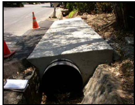
Photograph 43 (left). Lower open portion of Stewart Canyon Creek flood channel. Photograph 44 (middle). Fire-fighting activities that damaged aquatic habitats on San Antonio Creek. Photograph 45 (right). Example of undersized culvert for driveway entrance.
